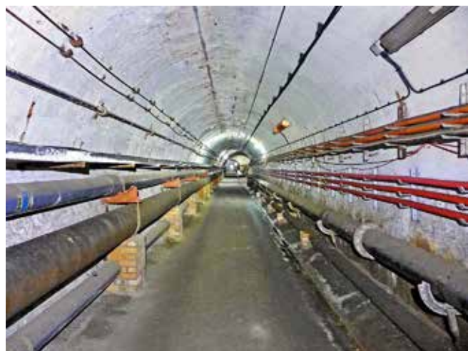
Admiralty Tunnel, the lined western end
